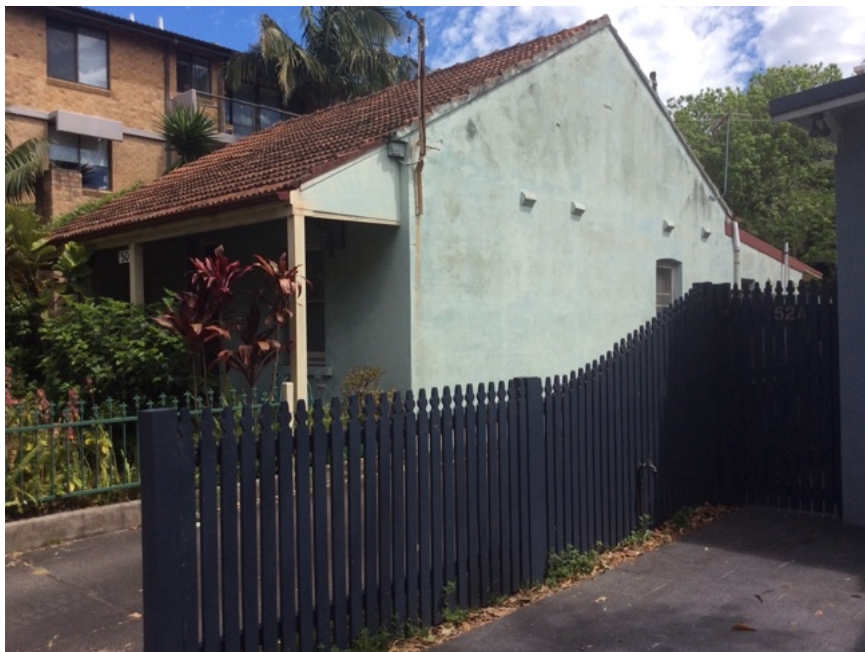
Figure 5: View of No. 50 Parraween Street. The roof form has been altered with the loss of the originally separate front verandah roof and recladding in unglazed terracotta tiles, which have caused inflexion in the roof (original roofing would have been either slate or corrugated iron, both lighter in weight).
